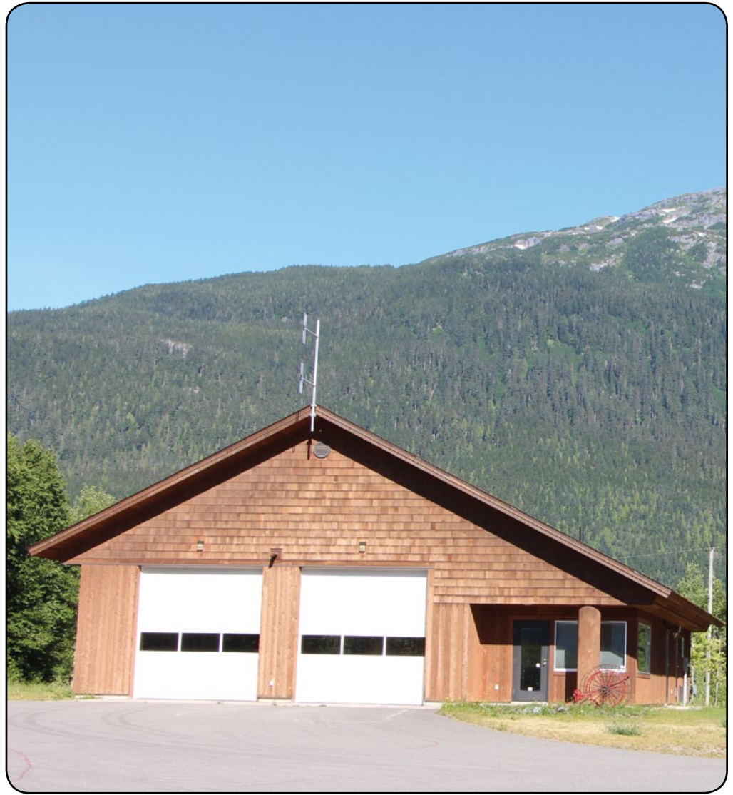
The Gitaus Fire Hall is one of three halls that are part of the Thornhill Fire Department. The other halls are in Terrace and at Lakelse Lake.
