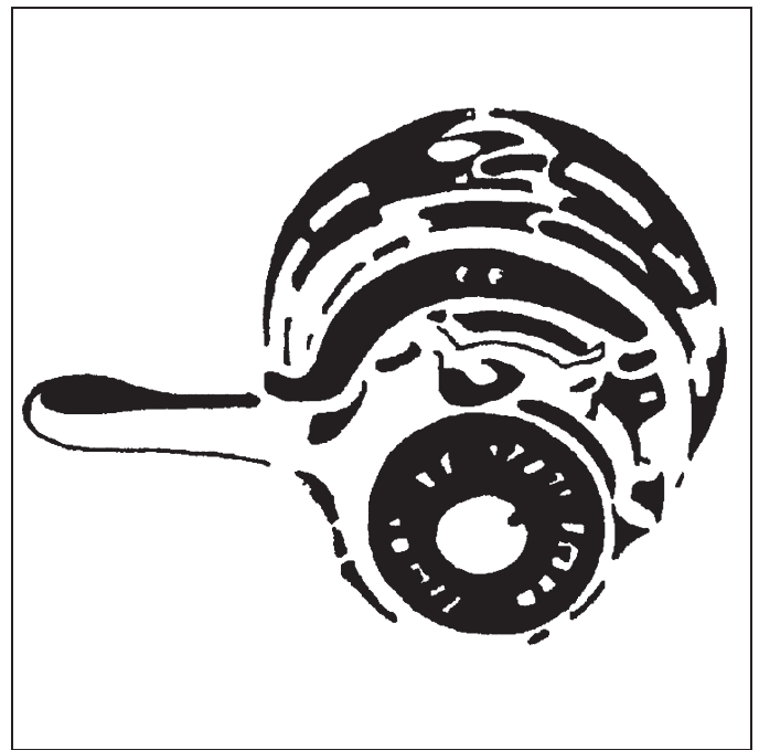
A single mixing control with a lever handle, for shower and bath, is easier for people who have difficulty grasping things.
